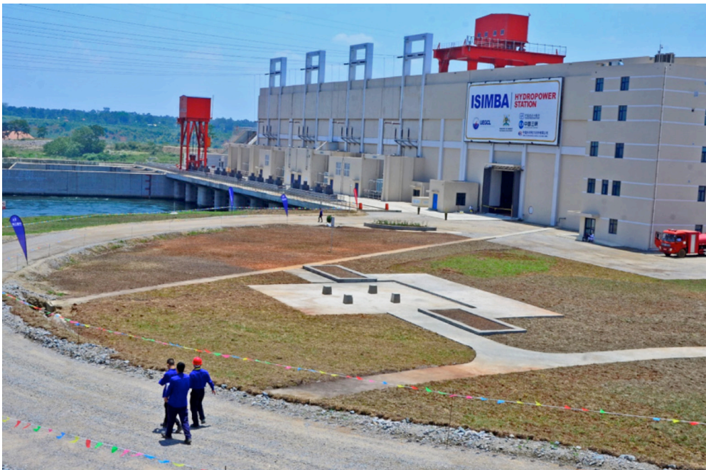
The newly launched Isimba Hydro Power Station in 2019. The project was delayed as well owing to varied reasons but prominently the unprecedented corruption allegations that rocked the process of compensation pointing out inflation of compensation rates by the office of the Chief Government Valuer. It took the intervention of the Commission of Inquiry into Land matters to halt this dubious payment.
